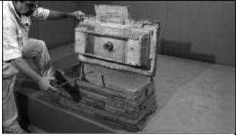
**2.** Mark position for water stub-up, minimum of 6" maximum of 20" from pool wall. Maximum 6" tall.
