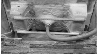
**4.** Plumb waterfall to stub-up using PVC glue (not included). We recommend that from the stub-up to the provided 1" female fitting, that flex PVC hose and a union be utilized (not included). Include an extra length of flex PVC curled up inside the waterfall so the Scupper can be drained or removed for the winter. The top of waterfall just snaps into position on top of the base.
