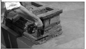
**3.** Once stub-up is installed, place Scupper over the stub-up and reposition to pool wall. Using 3/16" masonry bit and hammer drill, use the four provided locations as guides to drill holes for mounting screws. Screw in the provided blue Tapcon screws... tighten securely but do not over tighten.
